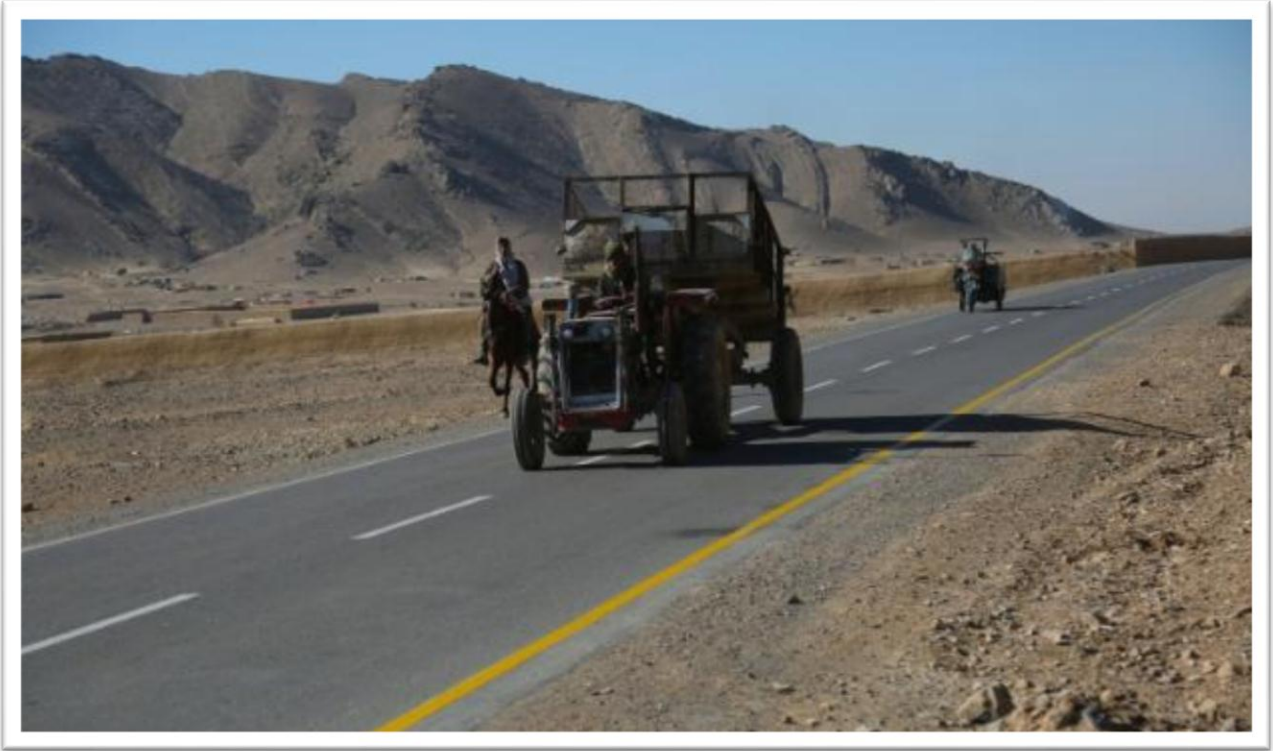
Construction of rural road in rural area provide access for transportation of local products
