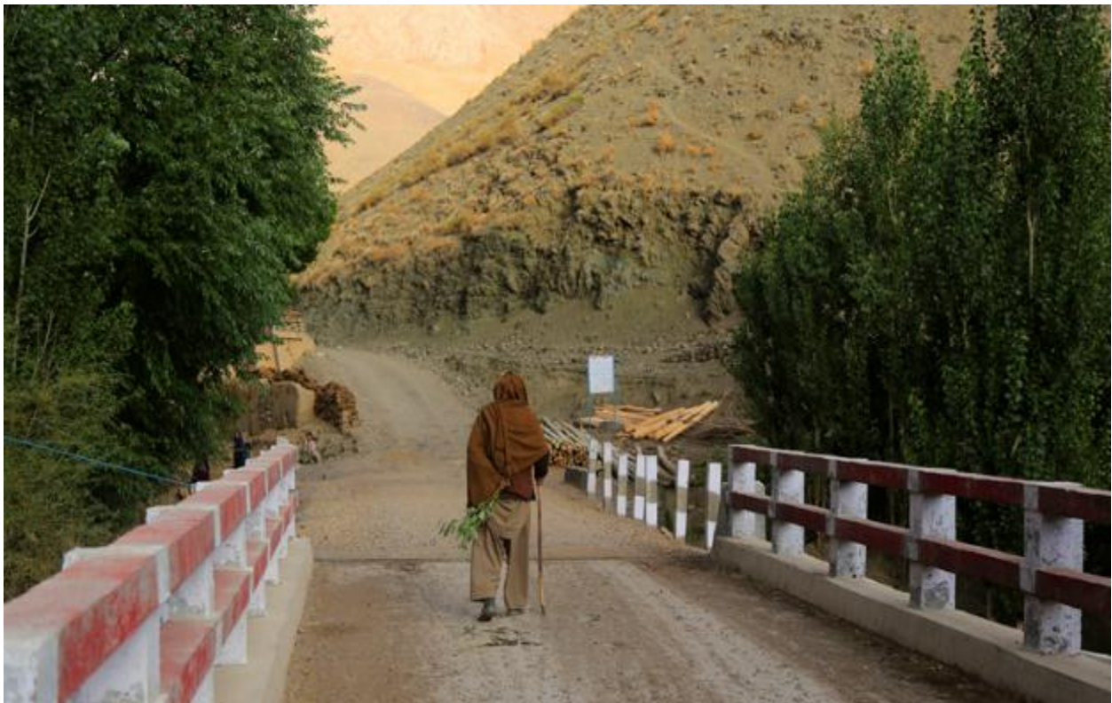
Construction of concrete Bridge in rural area provide access to transportation of local products
