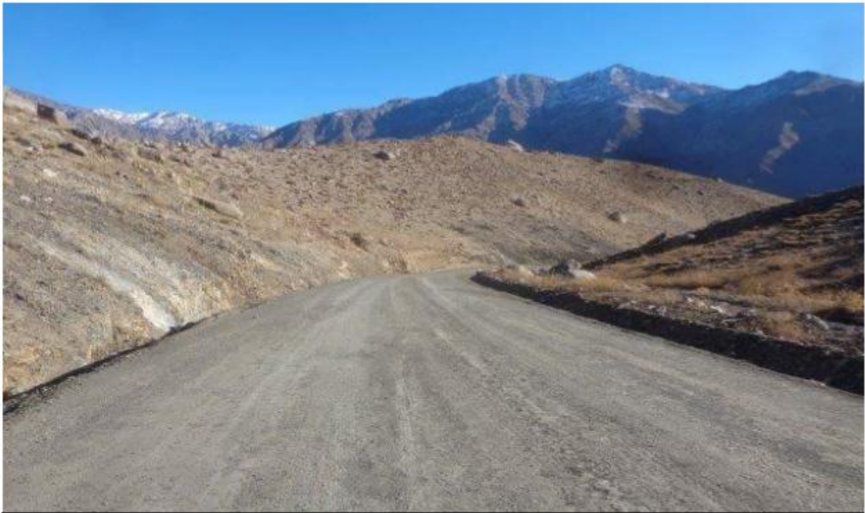
Construction of rural road in rural area provide access for transportation of local products
